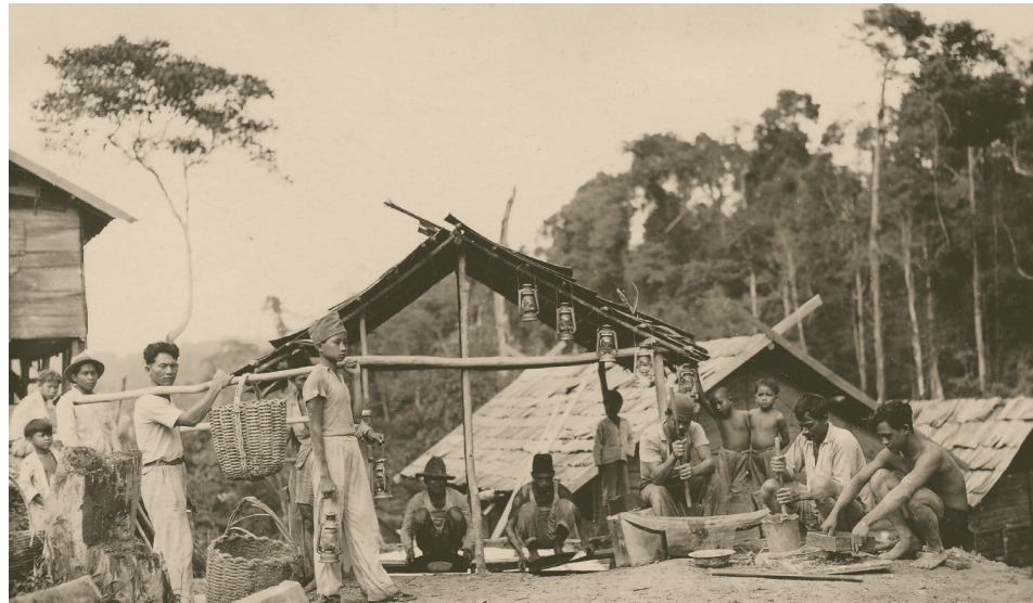
Fig. 2 Dayak goldminers bring ore to their houses where they grind and wash it, Tewah/Kalimantan, photo by Karl Helbig, 1937 (Roemer- und Pelizaeus-Museum Hildesheim).
