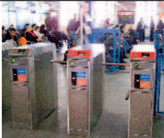
Abb. 6 Zugangskontrolle per elektronischem Ticket am Fähranleger in Istanbul (03/2007) Access control by electronic ticketing at sea taxi landing stage in Istanbul (03/2007)
