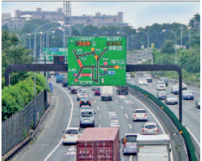
Photo 1 Variable graphic signboard
